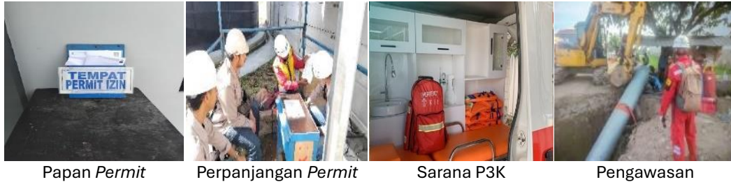
Gambar 4, Proses Hot Work Permit Sumber: Data Primer, 2024
